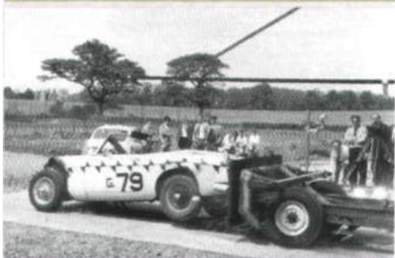
BGT Rear impact trolley (same weight as car).
